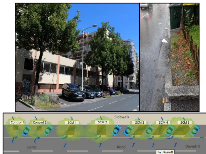
Figure 1. Study site. Left: Stormwater Trees. Right: Stormwater tree's infiltration trench during a rainfall event. Bottom: schematic top view of the site.
